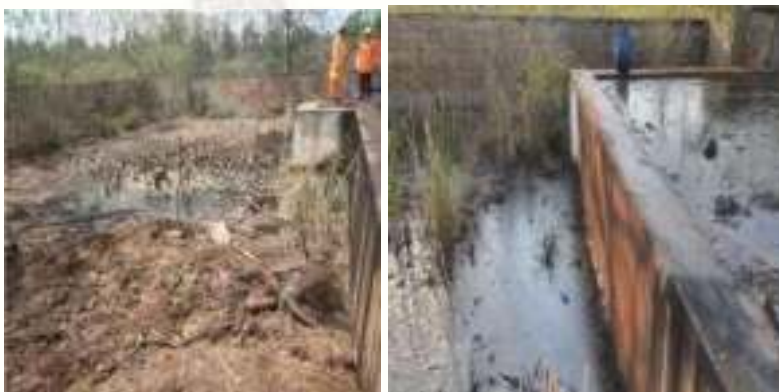
Photo 9: area surrounding the sludge tank
