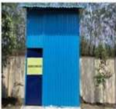
Photo 3: Hazardous waste storage shed
