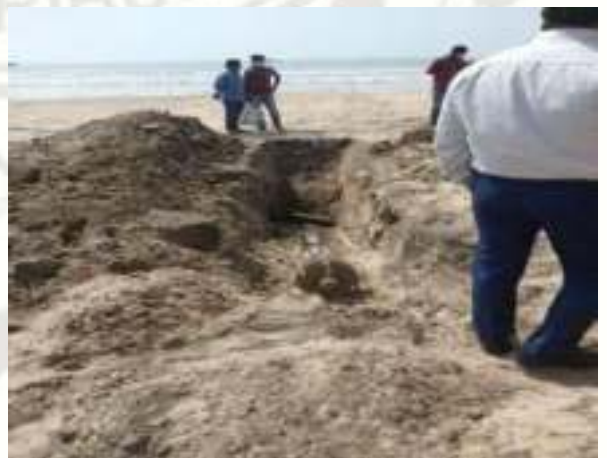
Photo15: laying of new pipeline
